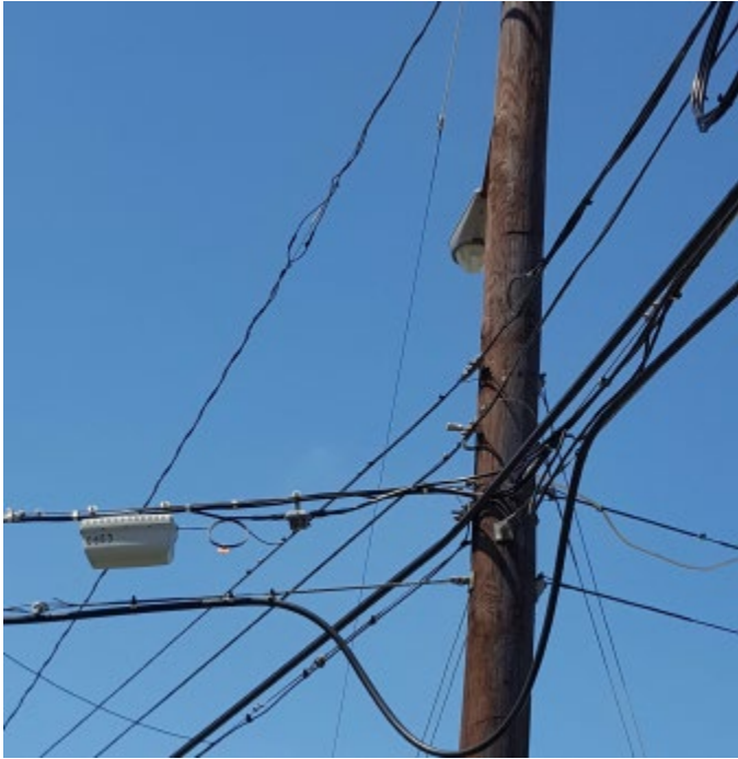
Comcast strand-mounted WiFi access point
